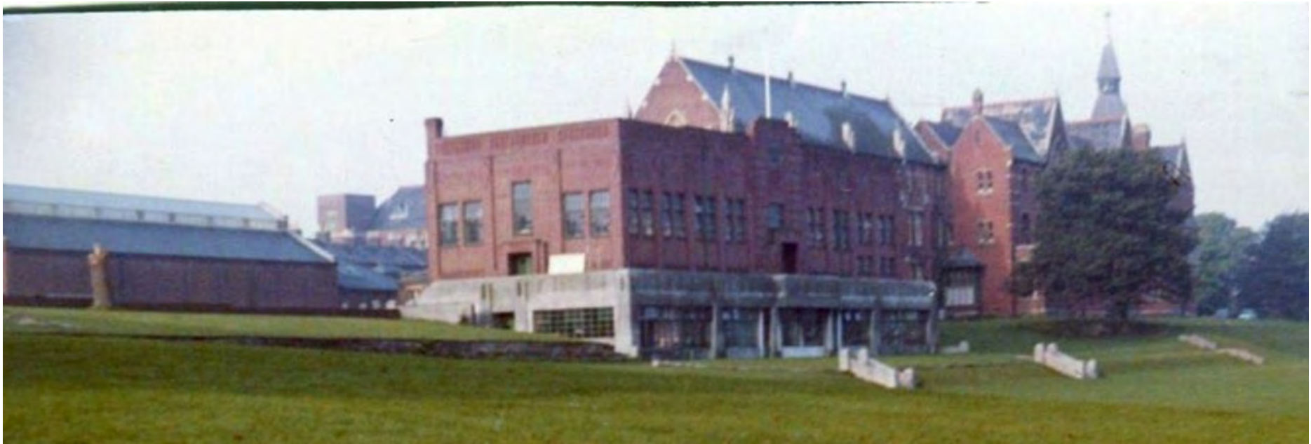
Plate 8: View of the school from the playing fields prior to demolition (facing WSW)
