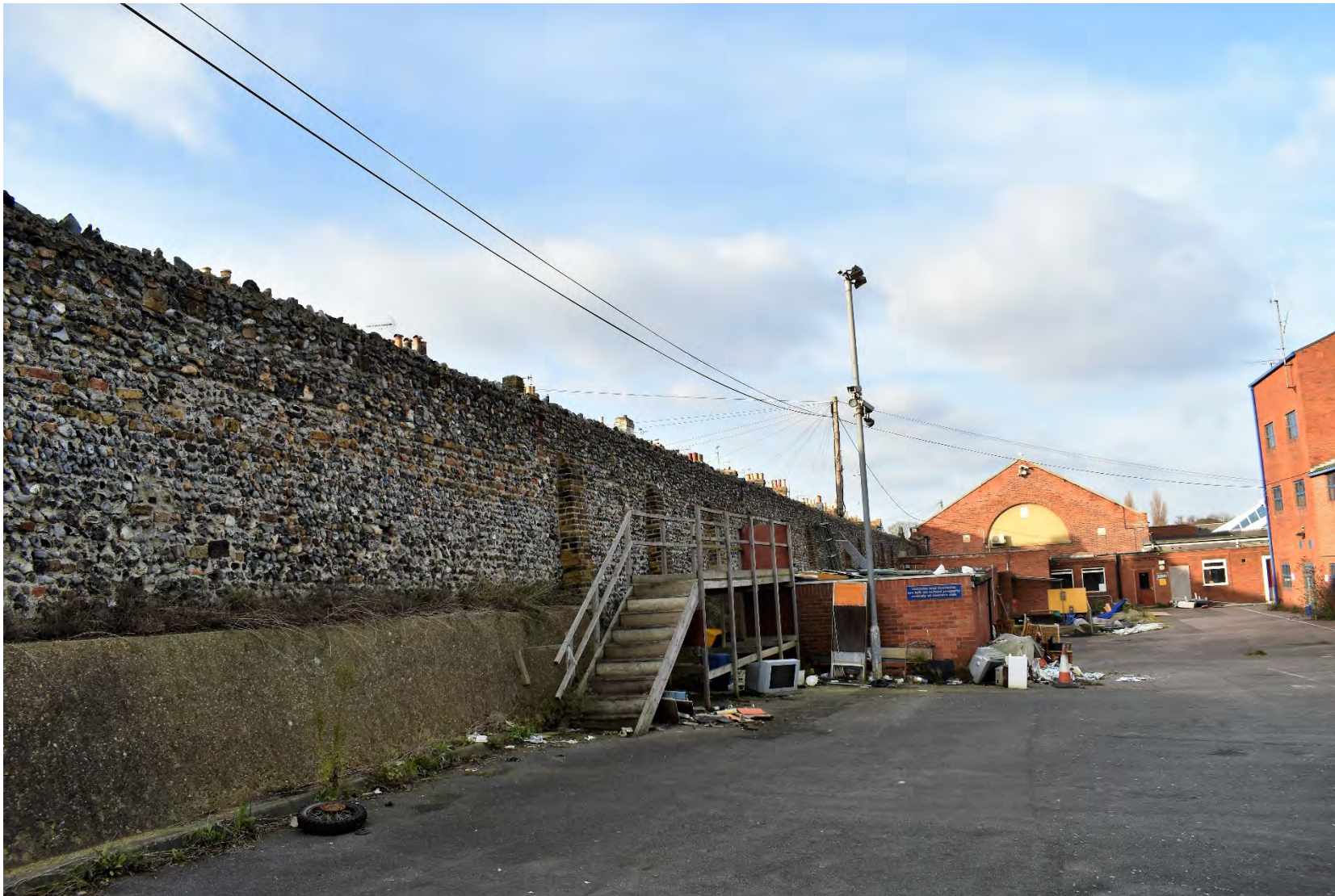
Plate 19: the northern side of the Bungaroosh wall within the school area (facing SW)
